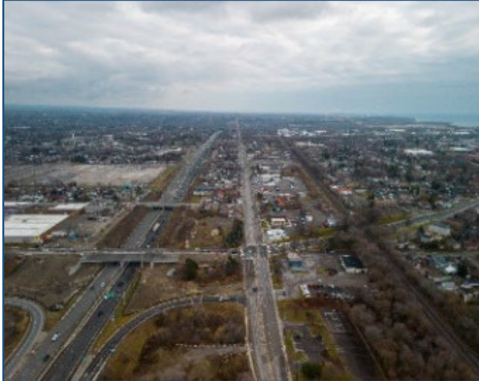
Figure 10: Photo of the Bloor Street and Simcoe Street South intersection, facing east
