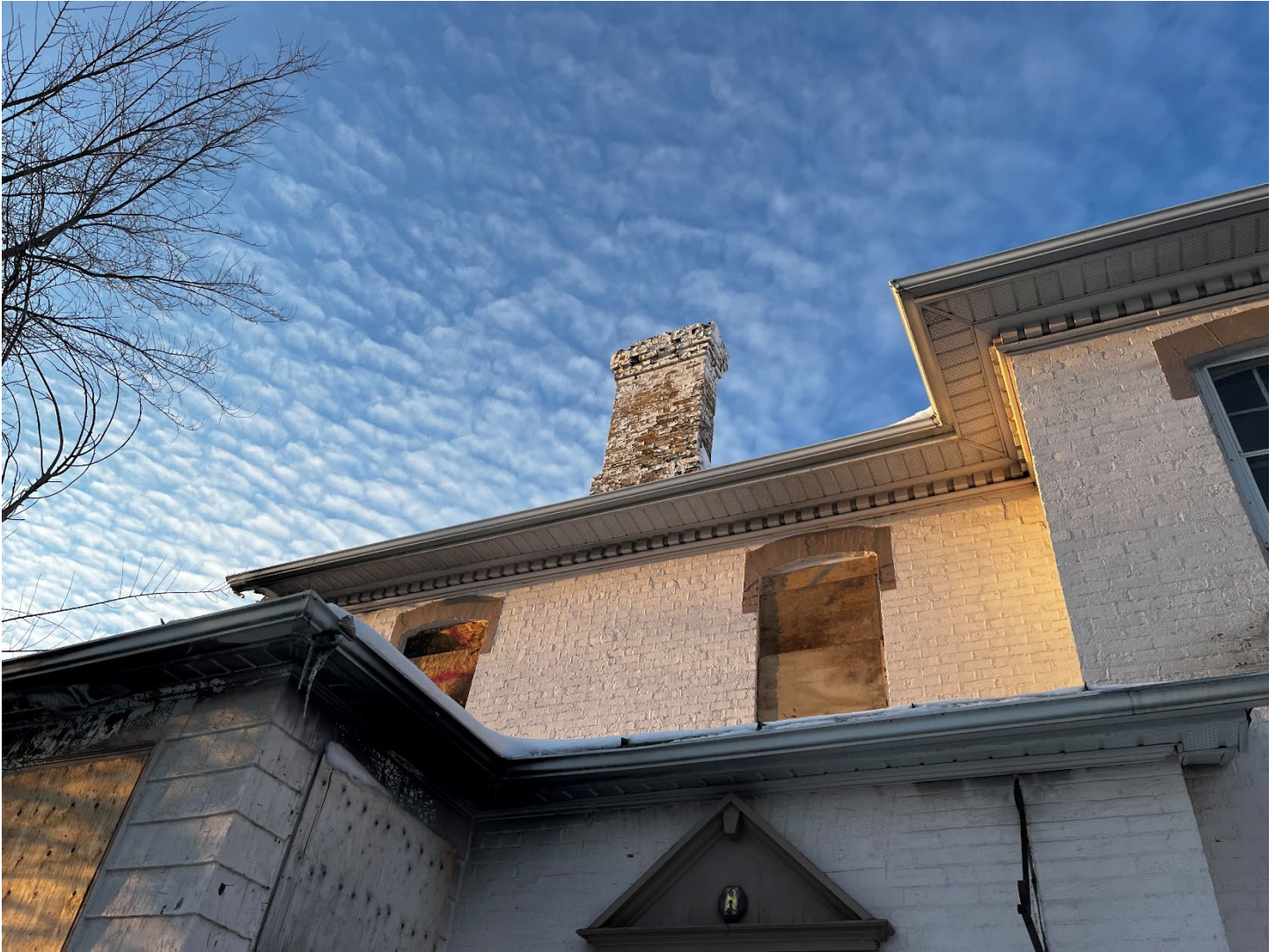
Figure 8 - Deteriorating chimney with potential for restoration
