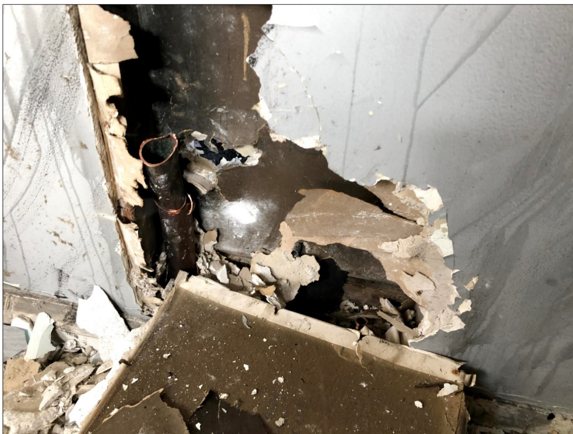
Figure 15: View of smoke impacted interior wall cavity in southeast bedroom (Sample B-6) on second level
