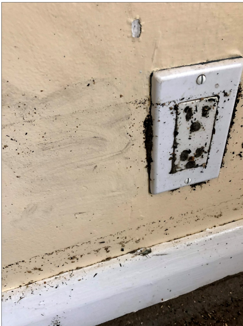
Figure 9: View of electrical socket plugged with debris
